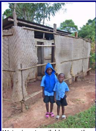
Water is not available near the latrines for washing hands
