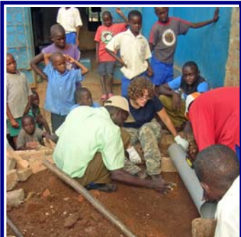
Christa lays out drainage pipe
