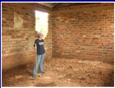
Christa leveling a classroom floor with rock
