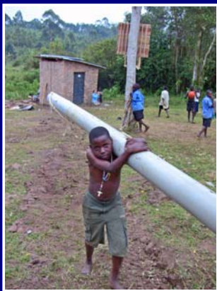
Hauling PVC well casing
