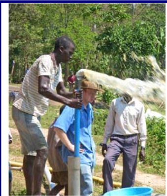
Developing the well using PVC pipe with a check valve on the end
