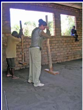
Melissa and students compacting the base layer of concrete
