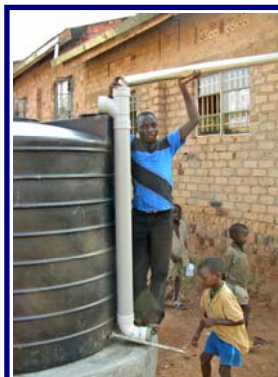
The roof catchment system with a first-flush bypass
