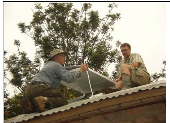
Bill and John on the roof making the final installation of one of the assemblies. Panels are installed horizontally at the equator
