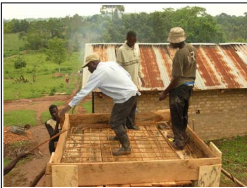
Placing the reinforcing for the slab
