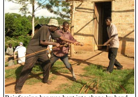
Reinforcing bar was bent into shape by hand
