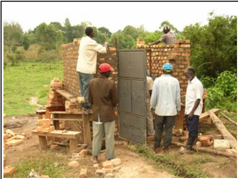
Volunteers constructing the generator house
