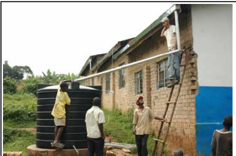
Dave inspecting the final roof catchment system
