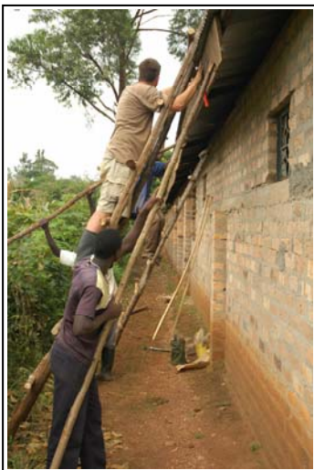
John installs lumber structural supports for the gutters
