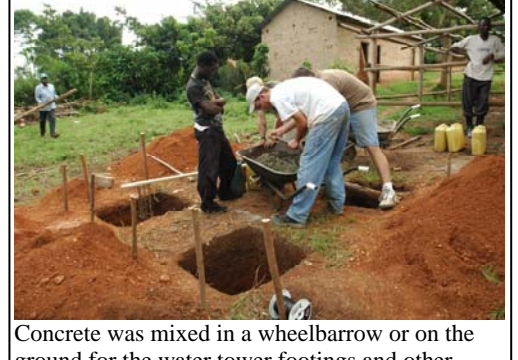
Concrete was mixed in a wheelbarrow or on the ground for the water tower footings and other construction
