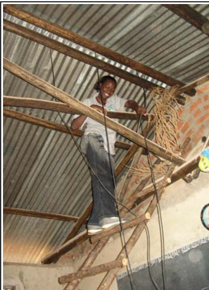
Violet feeds wires from the solar panels through the roof and helps with the interior wiring. The volunteers learned important new skills during the project
