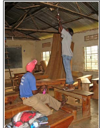
Peter (one of the teachers at the school) and Violet install lights in one of the classrooms
