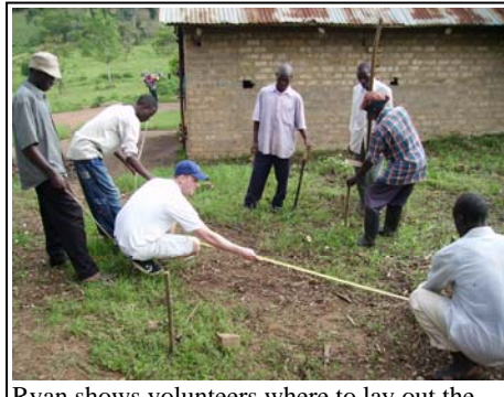
Ryan shows volunteers where to lay out the footings for the water tower
