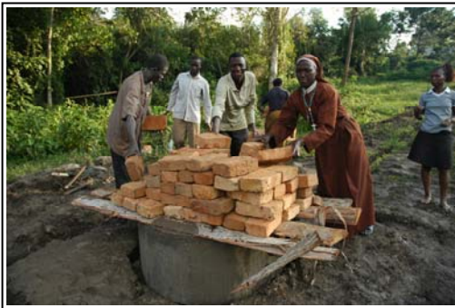
Well cylinders were weighted with bricks overnight to make them settle faster
