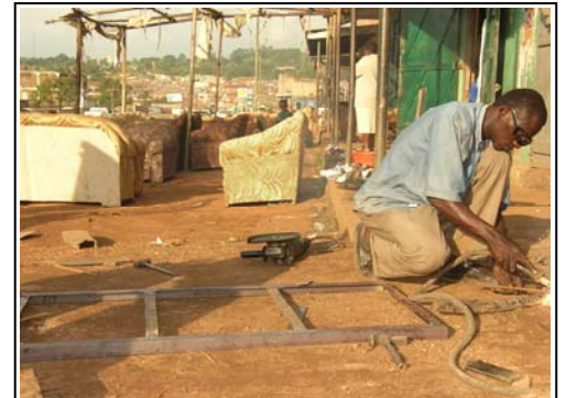
Fabricating the frames for the solar panels at the metalworking shop
