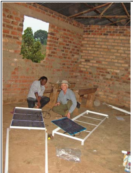
Bill and Violet (a Ugandan college student volunteer) installing the solar panels into the painted frames. This is in one of the school classrooms
