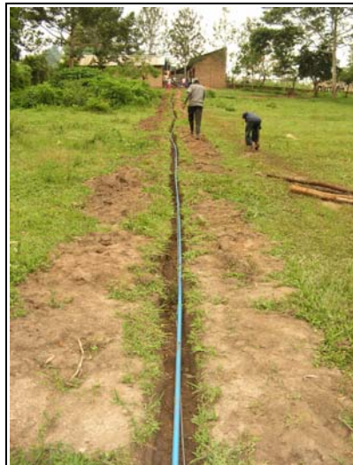
The 260 foot PVC pipeline connecting the well and the water tower was completed in two days
