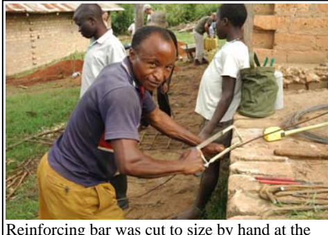
Reinforcing bar was cut to size by hand at the school
