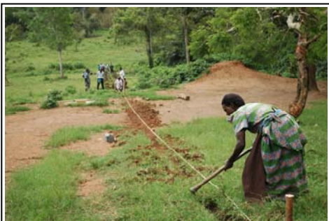
Digging the trench for the pipeline began on the second day
