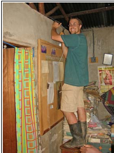
John installs wiring for the interior lights
