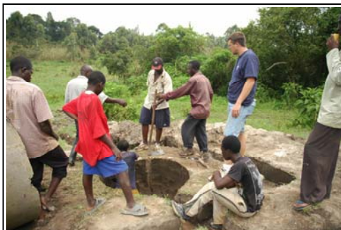
John supervising the start of the digging for the well
