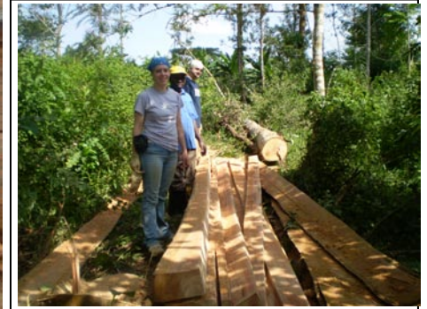
Lumber for the roof trusses and other construction was cut using a chain saw from eucalyptus trees on the orphanage property.
