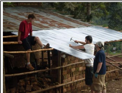
Evan and Tomas assist while Dan nails a roofing sheet over a shed area to provide additional shelter space for teaching the pre-school children.
