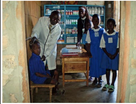
Looking through the new doorway into the examination area. The team installed new shelves for storing medicine. The shelves were stocked using funds donated by Interethnic Health Alliance in Salt Lake City.
