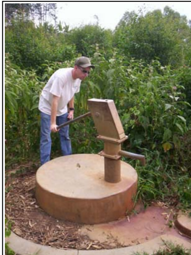
Josh tries a hand pump installed by others that doesn't work; another good reason why USU student skills and technical knowledge are needed
